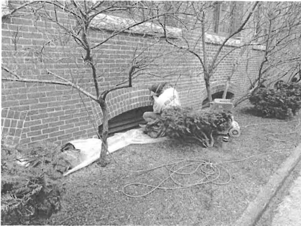
Photograph 3 – Workman cutting mortar joints in ground level masonry.
